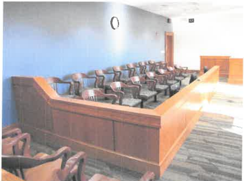
The expanded witness stand included a new low wall to match existing millwork, and new pedestal base chairs in the period style.
